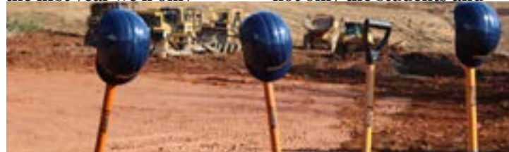
The equipment is set up and ready for the dignitaries to break ground.
